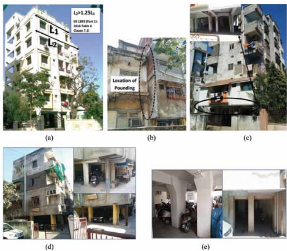
Figure 6. ((a) Vertical setback, (b) Possible location of occurrence of Pounding, (c) Overhang in form of jutting out balconies, (d) Poor quality of construction (e) Retrofitting through Column jacketing and steel I beam).
