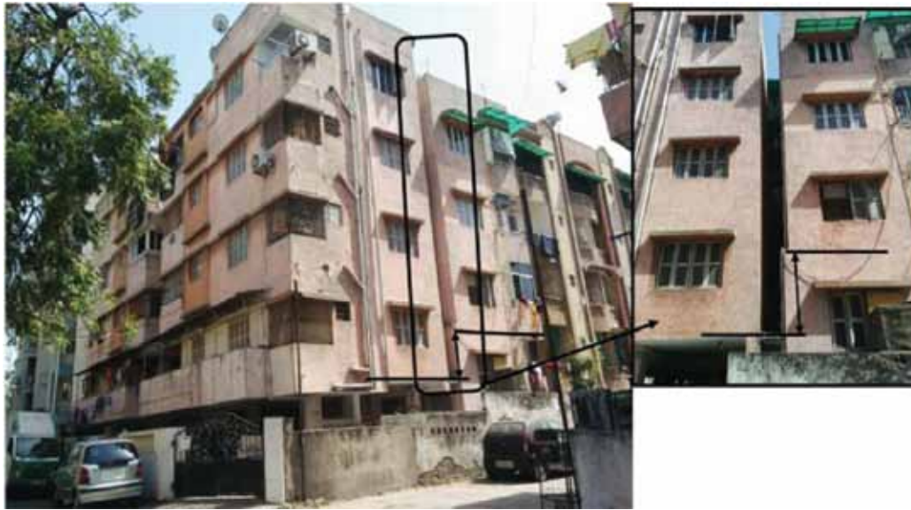
Figure 5. Partial soft storey
